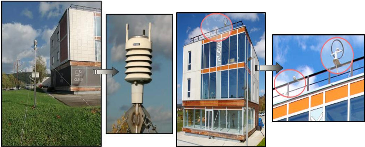
KUBIK's Local weather station and Solar radiation meters
