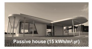
U<sub>walls</sub> = 0.32 W/m<sup>2</sup>.K Natural ventilation 0.4 ACH Infiltration 0.2 ACH
