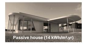
$U_{walls} = 0.09 \text{ W/m}^2.\text{K}$ Mechanical ventilation 0.4 ACH ( $\eta = 0.8$ ) Infiltration 0.07 ACH
