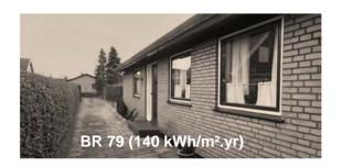
U<sub>walls</sub> = 0.32 W/m<sup>2</sup>.K Natural ventilation 0.4 ACH Infiltration 0.2 ACH
